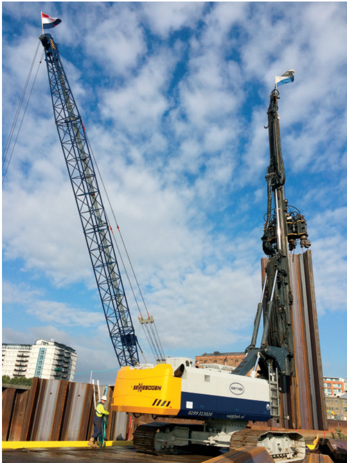
Silent Piler with quadruplet sheet piles
